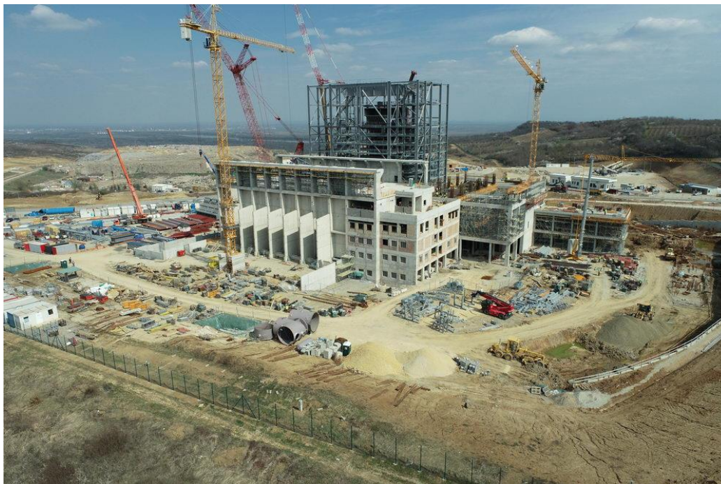
Construction of waste-to-energy facility at Vinča. Source: Beo Čista Energija
